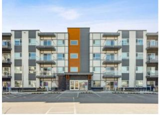
Cement Fiber Board, Concrete, Wood Frame
